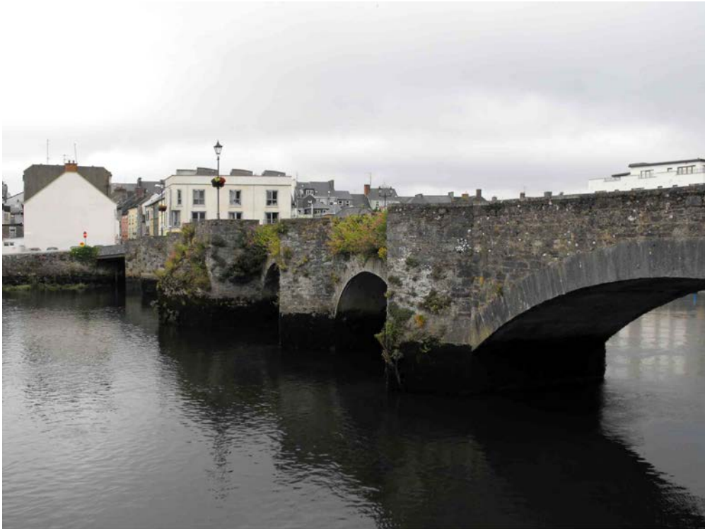
Fig 29 Carrick Old Bridge
